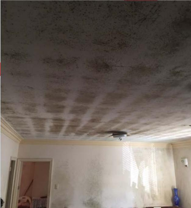
*Mould is an increasing problem in all buildings and constructions. Tightly built houses, together with insufficient ventilation, incorrect weather shields or water damage create mould growth. Mould spores are all around us and often cause little inconvenience. However, when these mould spores come into contact with wet or moist surfaces they start to germinate and create health concerns.*
